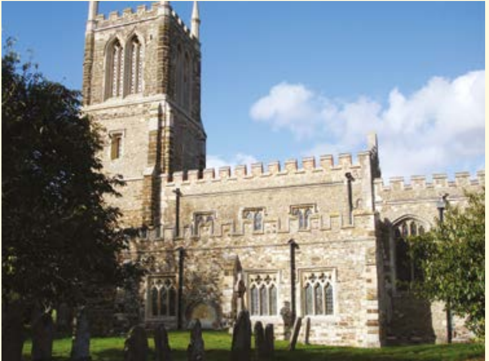
St. John the Baptist, Cockayne Hatley: Parapet repairs
