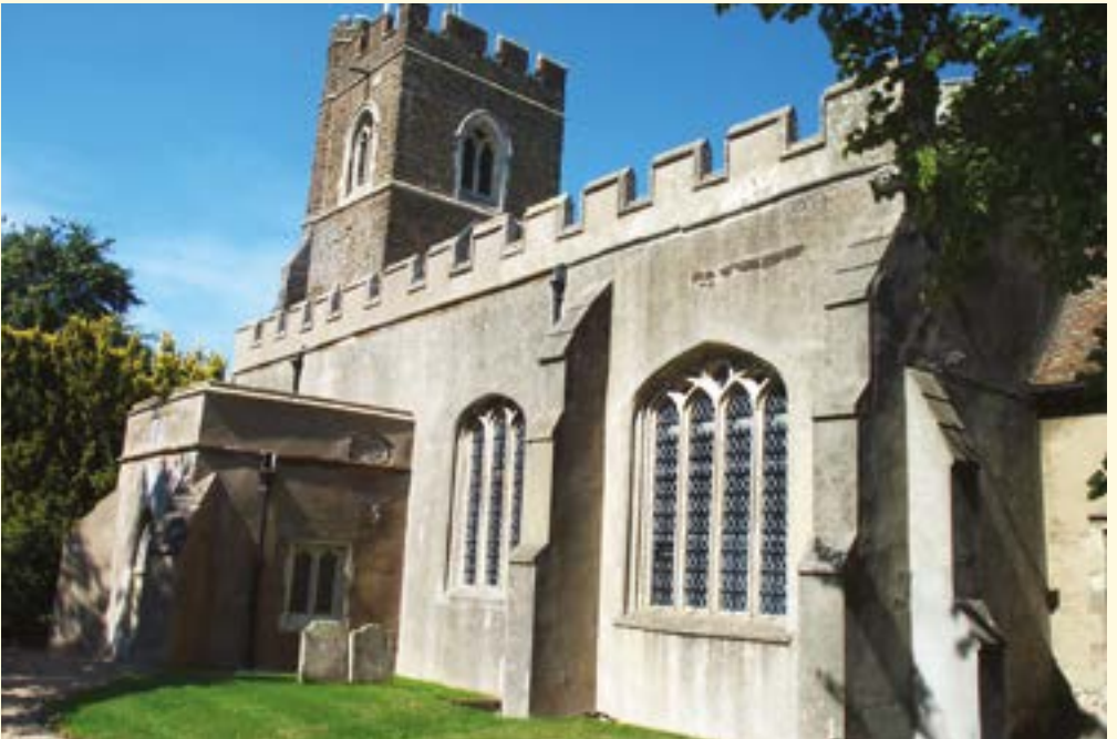
St. Mary Harlington: Porch and south aisle repairs
